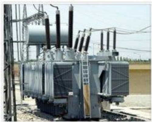
250MVA , 230/63kV transformer
