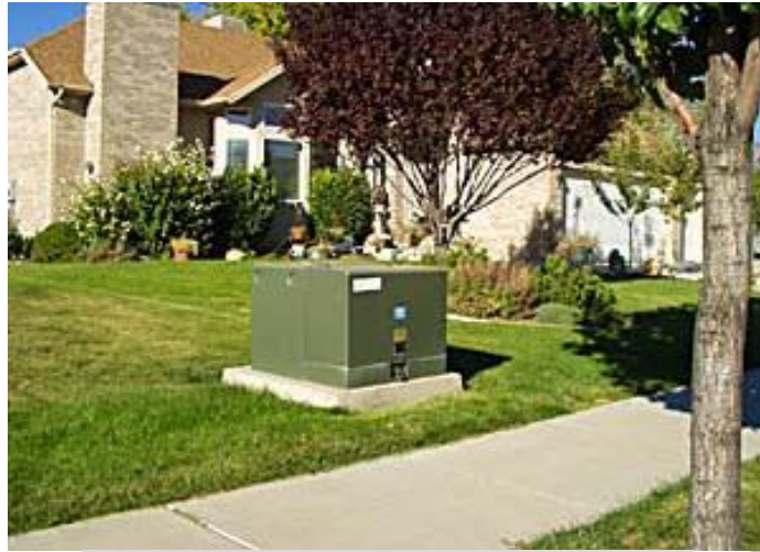
Residential - Ground - Transformer
