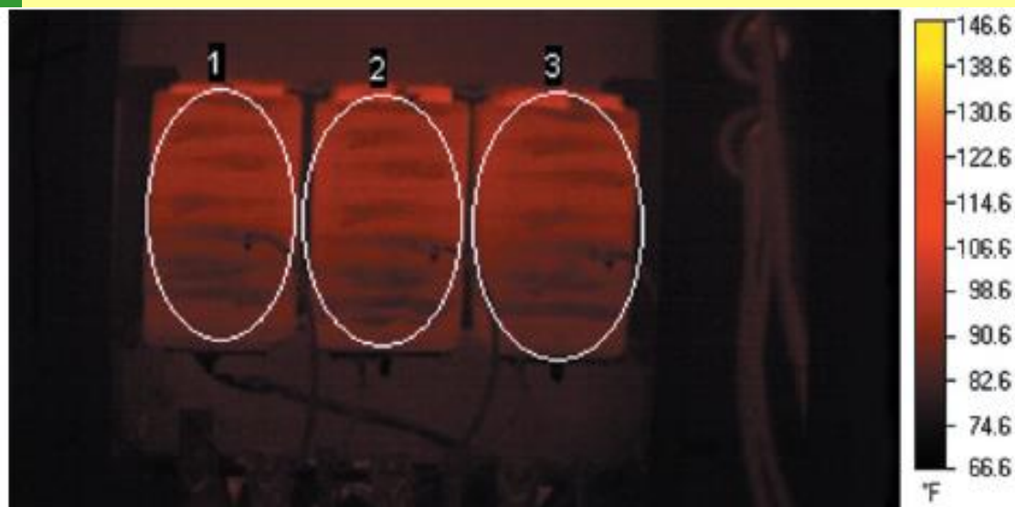
Photo 2 — Eaton's Harmonic Mitigating Transformer
